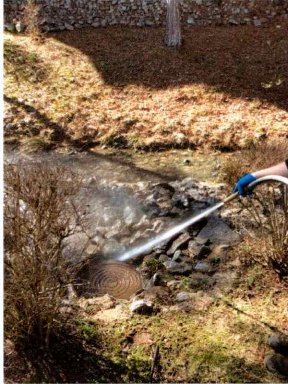
MH 3728 During cleanup
