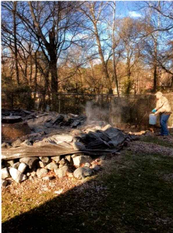
MH 1866 During cleanup
