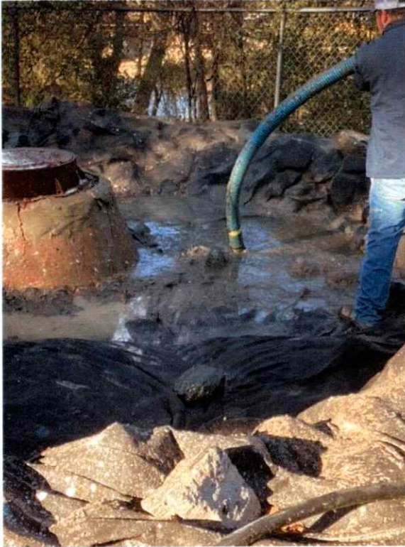
MH 1866 During cleanup
