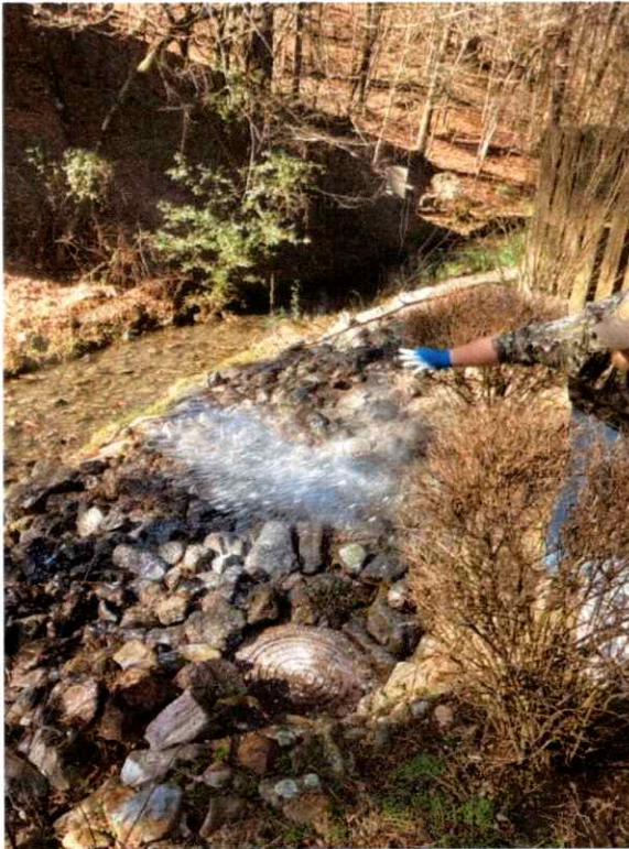
MH 3728 During cleanup
